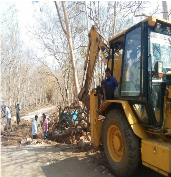
Installation of Pipe Culvert in Road
