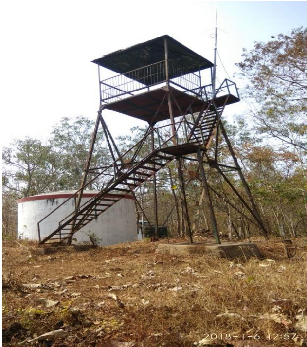
Repair of Watch Tower
